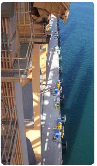
Following the success of trials carried out in 2005, the Port of Salalah installed four MoorMaster™ 600s at a berth servicing container
